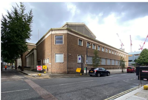
Picture 3: Views of the existing building from Sawyer Street looking West
