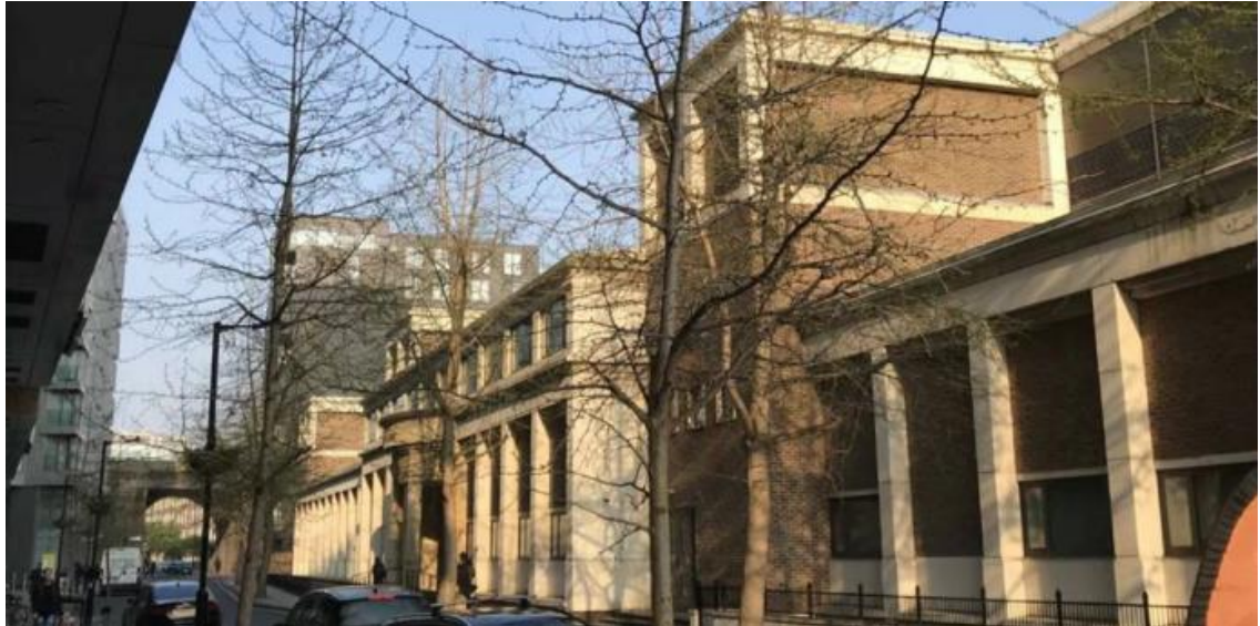
Picture 9: The Pocock Street elevation of the existing Crown Court building.
